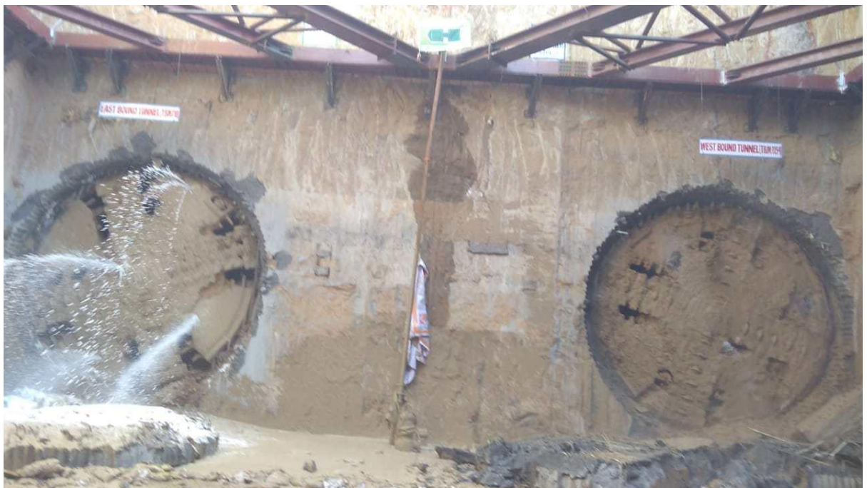
• 1st Twin Tunnel Breakthrough achieved by GMRC
