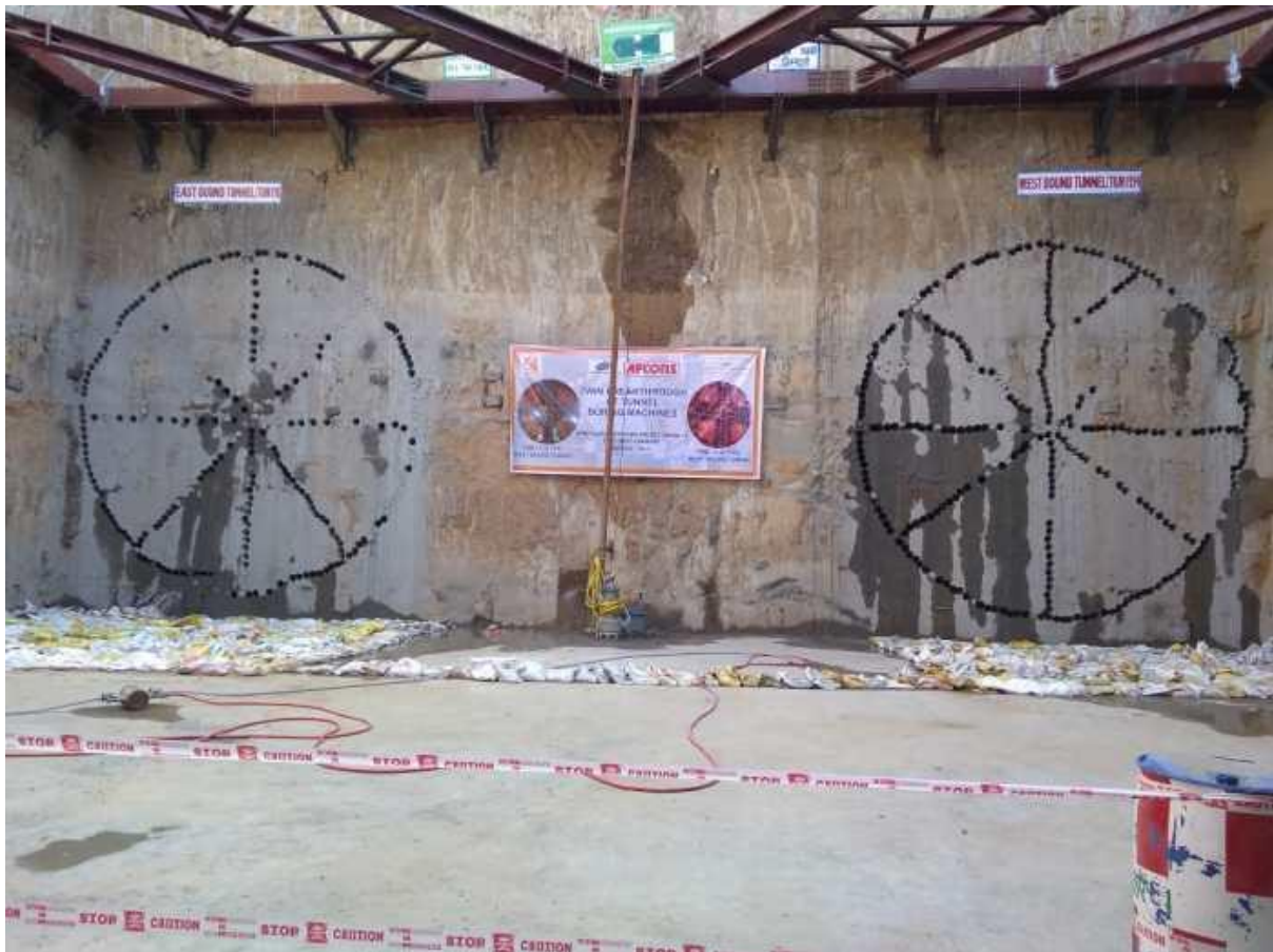
Ahmedabad Metro Achieve 1st Twin Tunnel Breakthrough at Kalupur Metro Station
