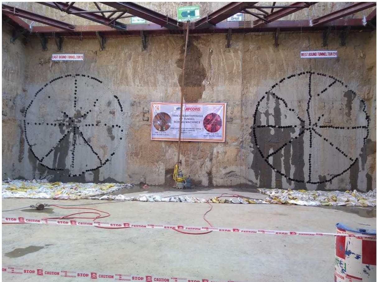
GMRC prepared for first twin tunnel breakthrough at Kalupur Railway Station
